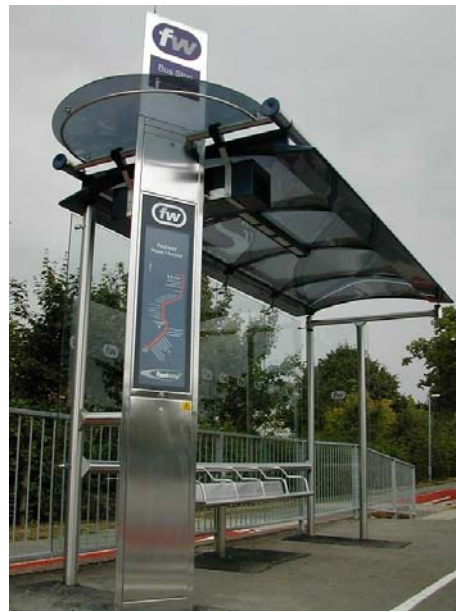
A number of Fastway bus shelters have been damaged since installation.
