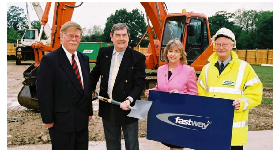
Cllr Doug Murdoch of Crawley, Lt Col Tex Pemberton WSCC Cabinet Member; Cllr Kay Hammond, Executive Member for Surrey join Site Manager David Uprichard at the start of works Fastway
